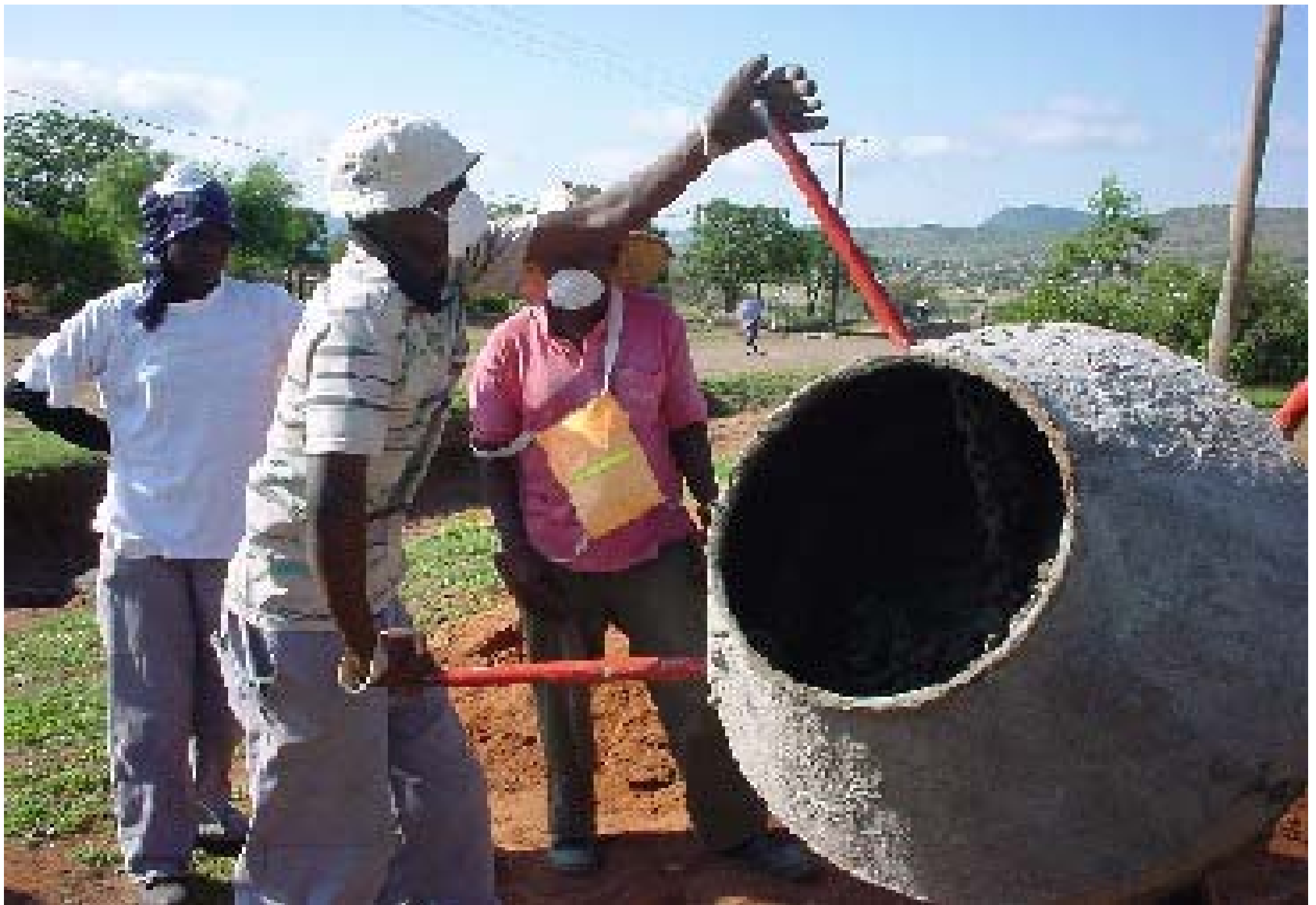
Mohlaletse, Greater Sekhukhune Hand operated Concrete Mixer
