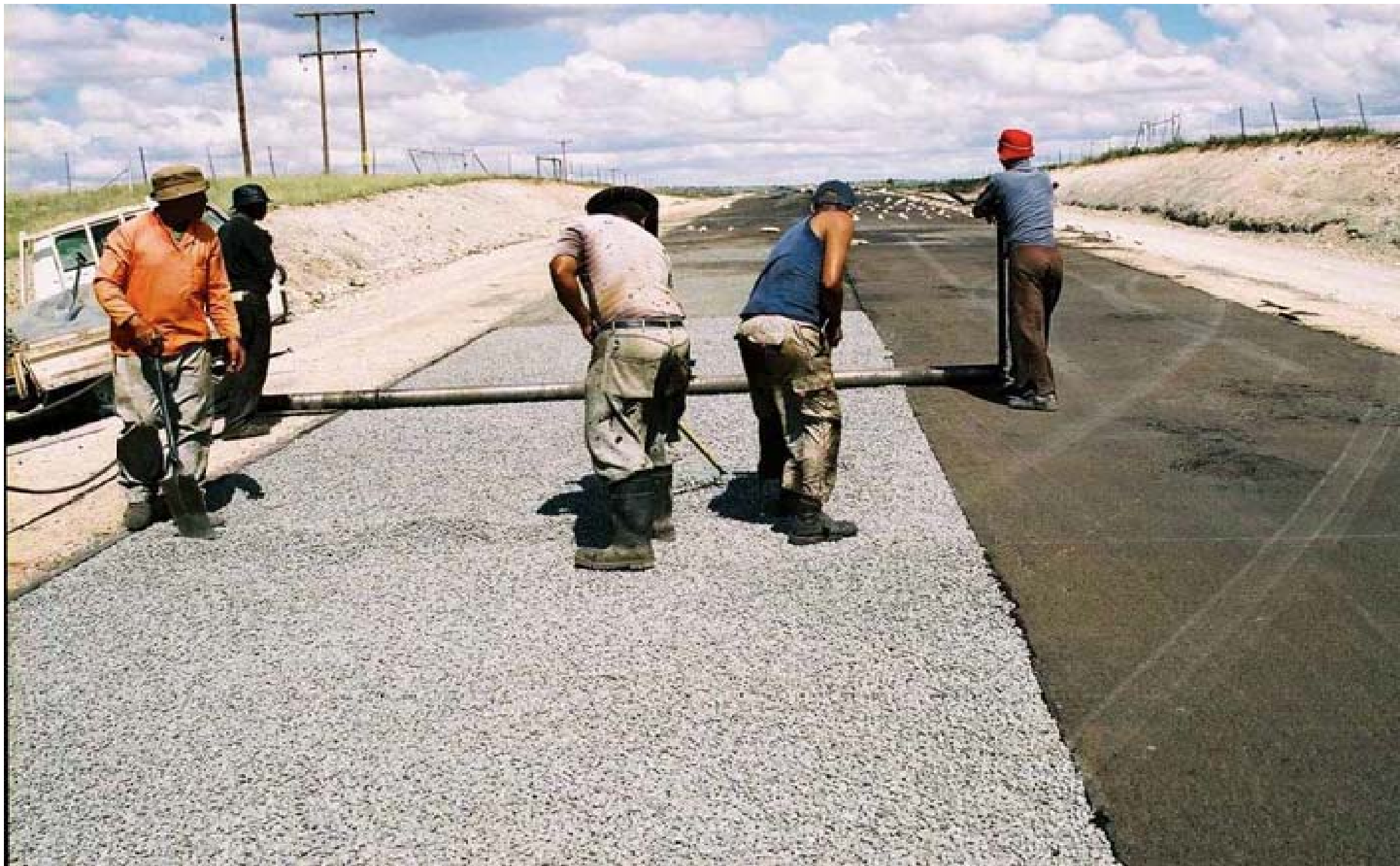
Provincial Road in Free State Province
