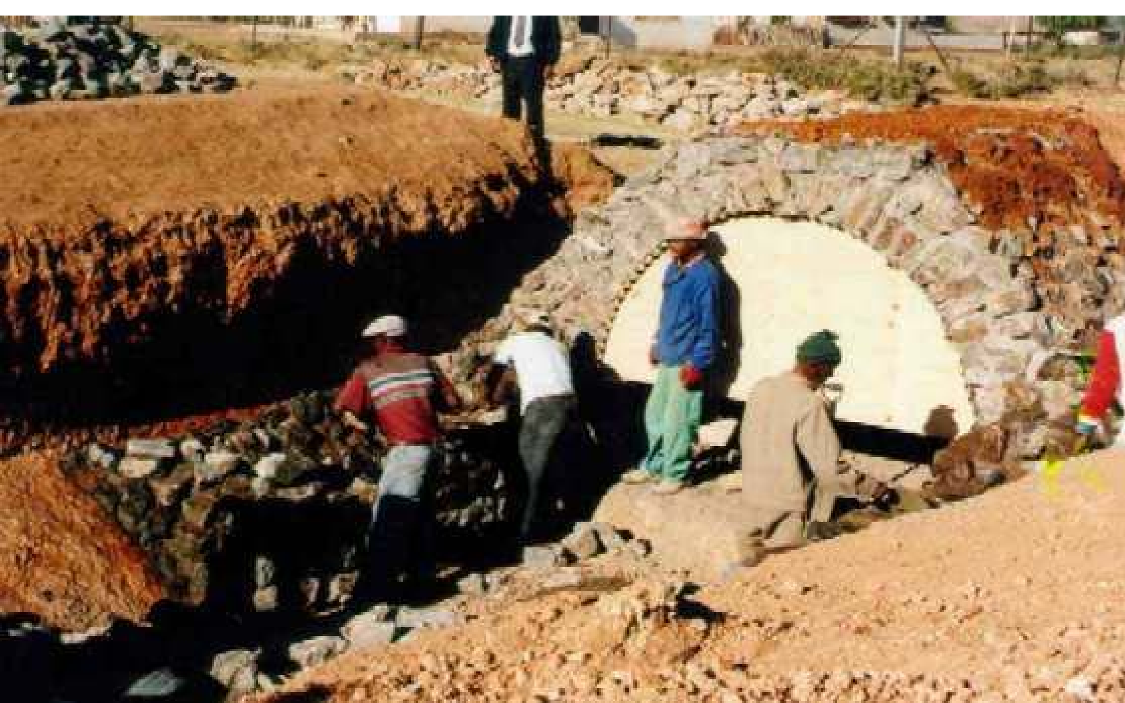
Sekhukhune: Rubble masonry culvert
