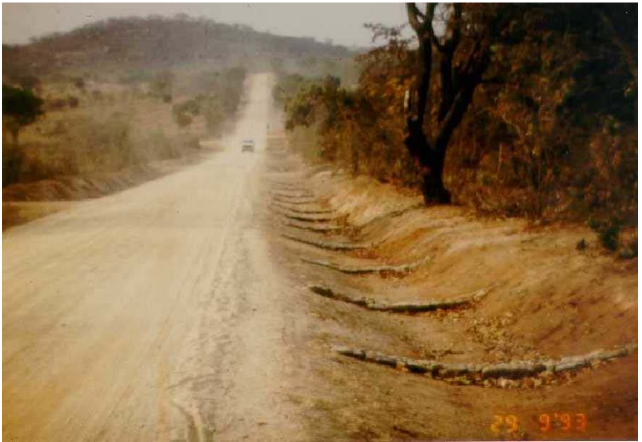
Zimbabwe: Based on techniques developed in Botswana this road is built to higher standards than those specified in Kenya
