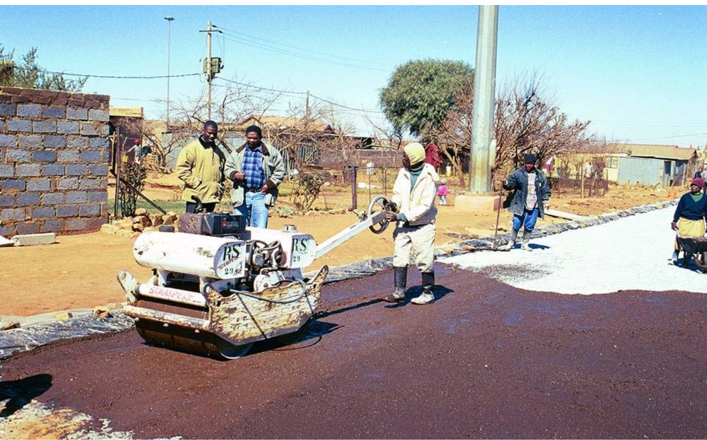
Bitumen emulsion in slurry bound base
