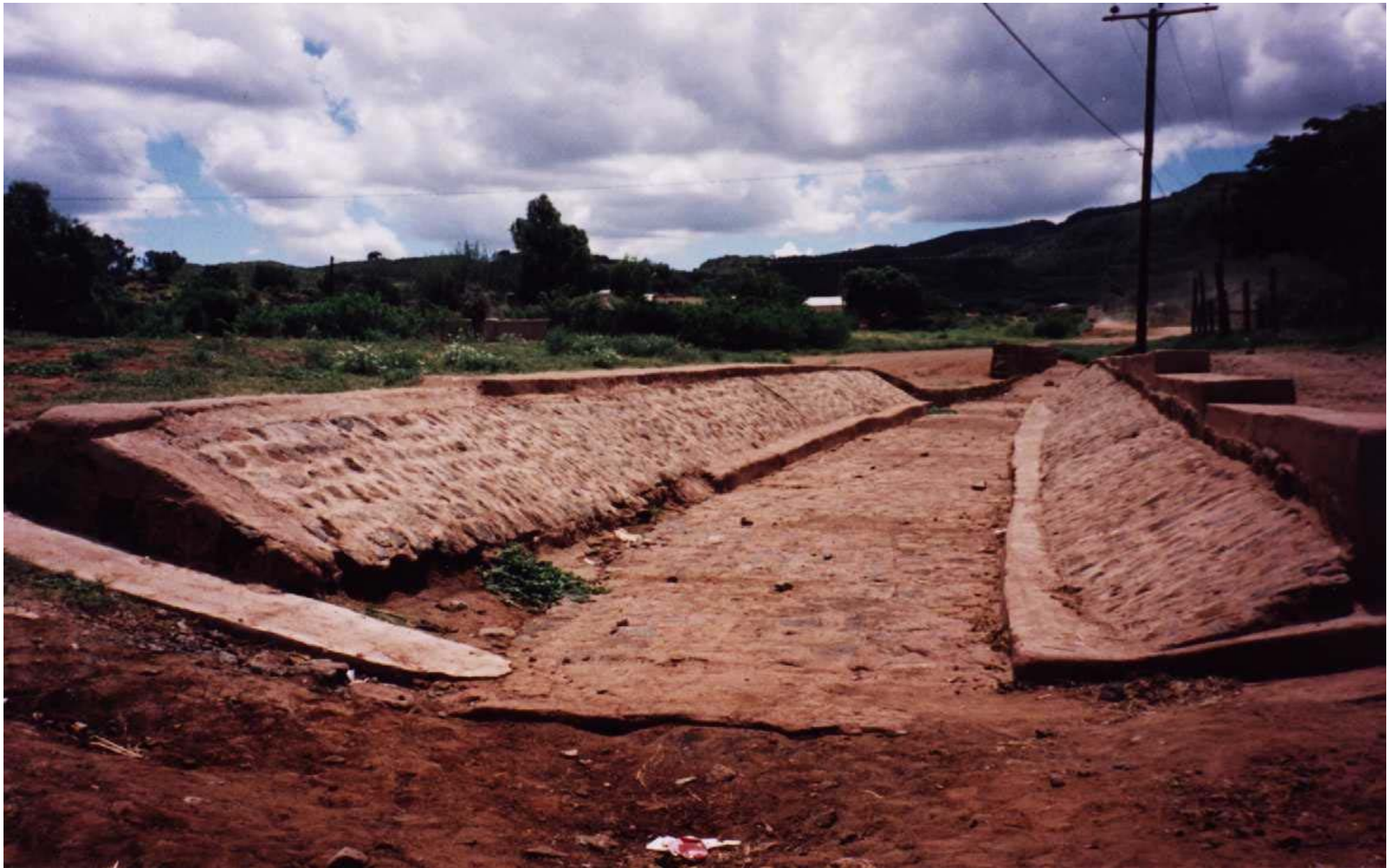
Mohlaletse, Greater Sekhukhune Stormwater Drainage (2)
