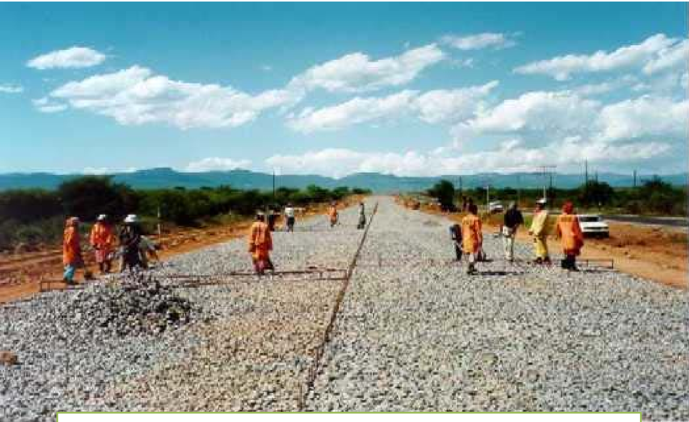
N 1 Matoks to Machado: WBM Base
